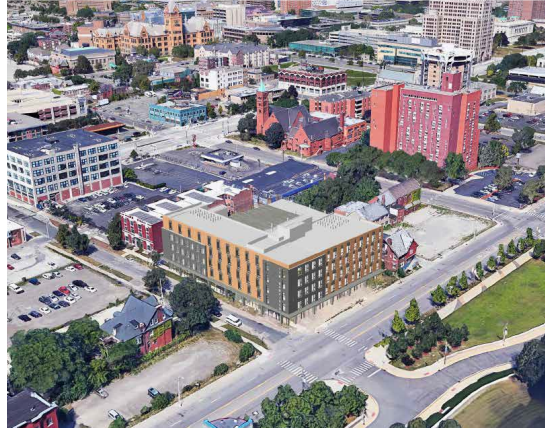
Sugar Hill Arts District Development, Midtown, Detroit Mixed-Income, Mixed-Use New Construction
